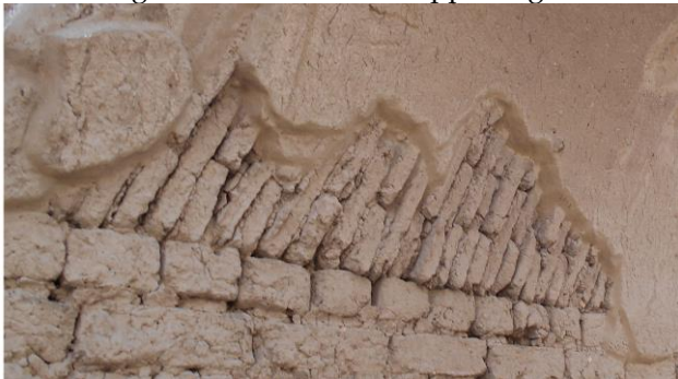
Figure 2 (Van Beck, 1987; Spencer, 1979). The inclination of the bricks from the vertical led most of the weight of each brick to transfer to the lower course which already had been laid rather than acting downwards, thus, the weight of each new brick was borne by those already laid. The brick was held in its position and stuck to the brick of the lower course by mud mortar.
