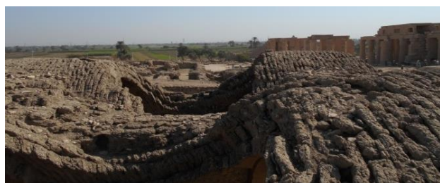
Figure 10. (a) The ruins of the Ramesseum temple and its storerooms vault and walls, (b) inside the storerooms.
