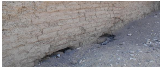
Figure 17. Holes made by wild bees after eating the straw in the plaster in the Ramesseum storerooms.
