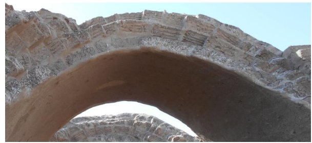
Figure 5. Bricks made with grooves to ensure the brick-mortar bond. The storerooms of the Ramesseum temple.
