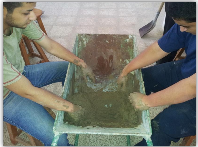
Fig. 9. Mixing the adobe by hand
